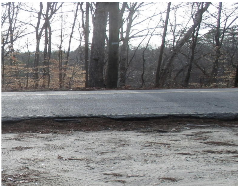
Figure 32: Pavement Drop-off
